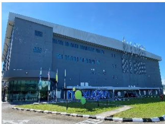
Novugen Pharma Manufacturing Facilities at Bandar Enstek Negeri Sembilan
